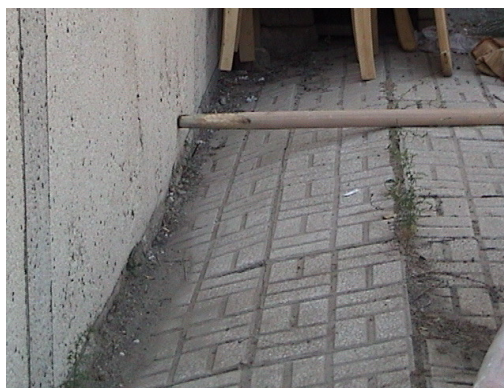
Fig. 1 Damages to flooring due to the swelling of gypsum soils
