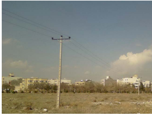
Figure 1- Cantilever reinforced concrete beam for transmitting electric power in urban environment
