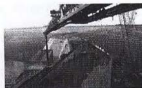
COVER: Placing RCC near the top of the Saluda Dam
