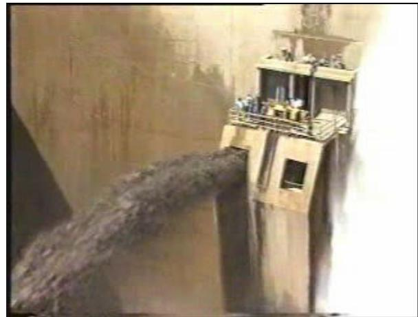
**Figure 2**- Pressure Flushing operation in Jiroft dam, Iran.
