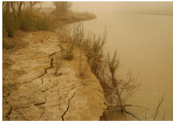
Fig 4: planar failure along with tensile cracks in the materials of Sistan River's bank
