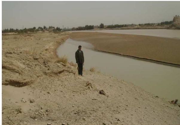
Figure 6. Sediment accumulation in the middle of the river channel
