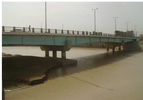
Figure 7. The accumulation of sediment on the site of hydraulic structures
