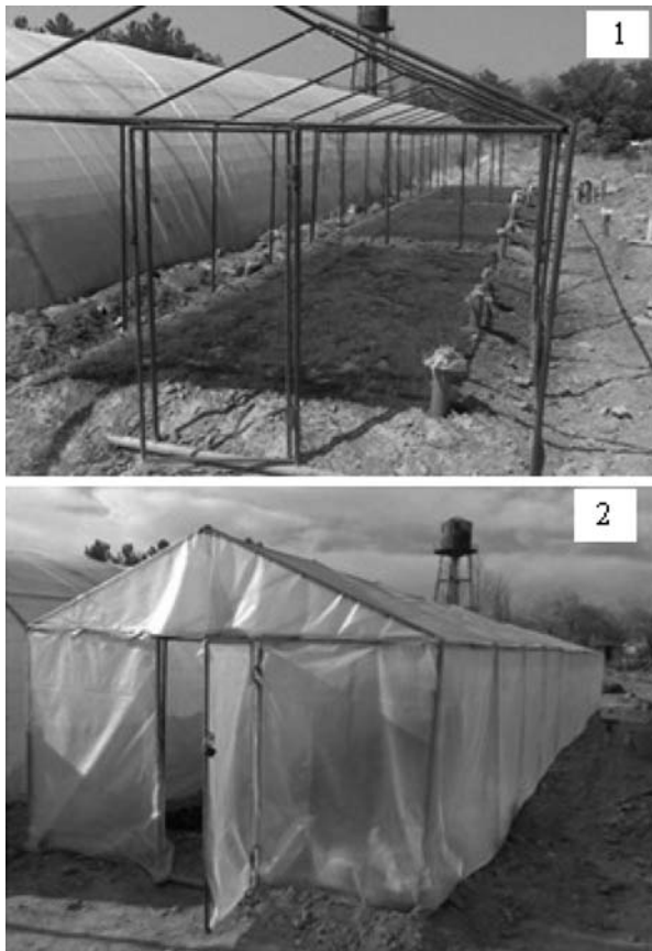
Figure 2. Metal frame with 100% vegetation coverage and the EAHE with inlets and outlets (1) and a greenhouse covered with plastic material (2).
