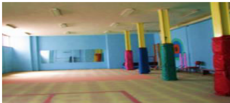
Figure 22: High school gymnasium in poor quality (Abnieh Tarrahan Alborz, 2008)
