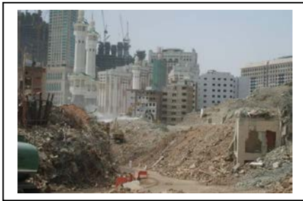
Figure 3: Demolition of historical fabric in Mecca Source: https://www.slideshare.net/brighteyes/mecca-construction-plans-for-the-future-kabah
