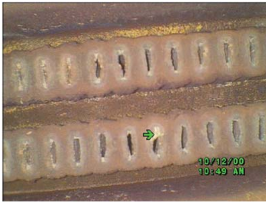
Fig. 3. Copper oxide deposits at the hollow conductor inlet [10]
