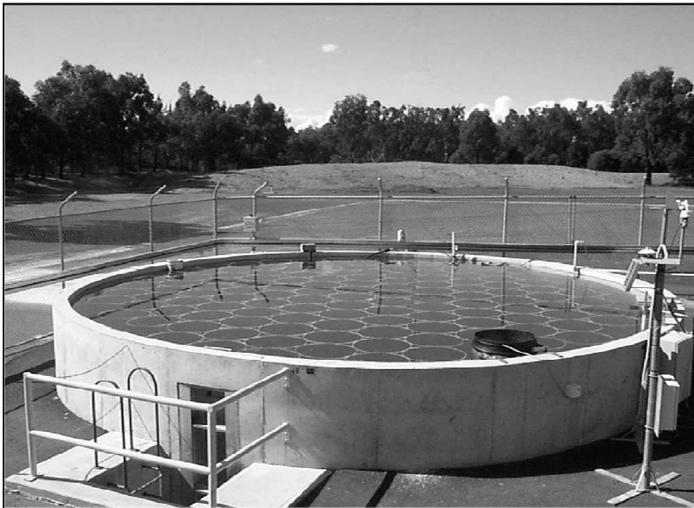
Fig. 1. (a) Schematic view of the pond with three zones, salt charger and surface washing system. (b) RMIT solar pond at Bundoora: the presence of the window (Eastward) facilitated the visual observation of water clarity at different depths. Floating rings and salt charger are clearly shown in the picture.
